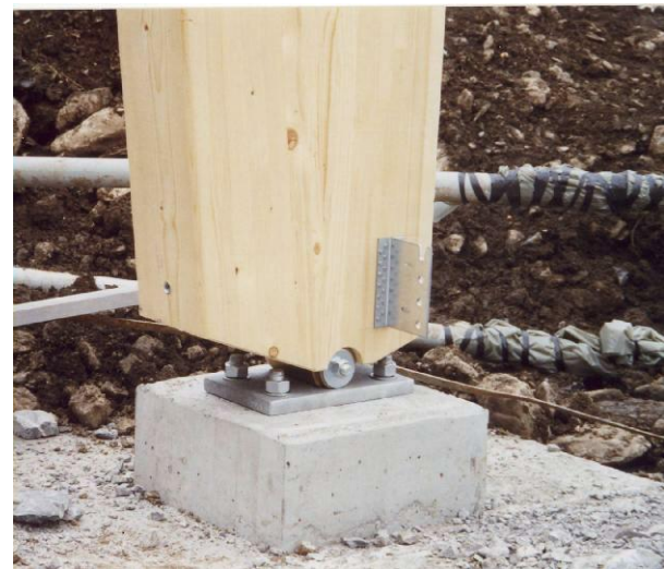
Figure 9: Pivot hinge in GSA®-technology
